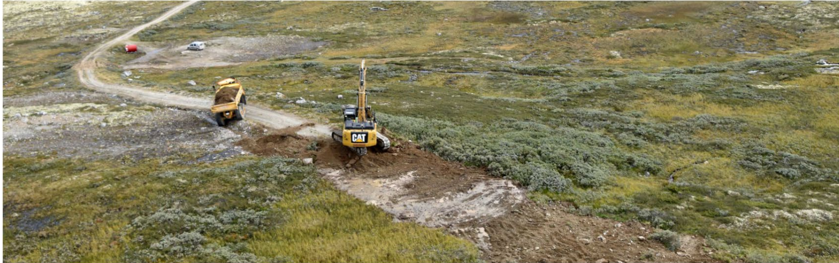
Road removal in progress. Photo: Dagmar Hagen / NINA
